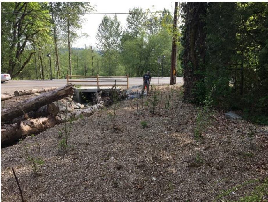
Anti-Aircraft Creek Culvert Located under Newport Way NW
