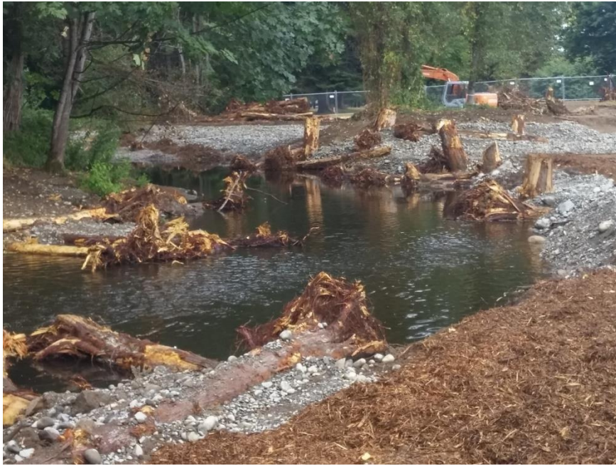
Expansion of Floodplain at Confluence Park
